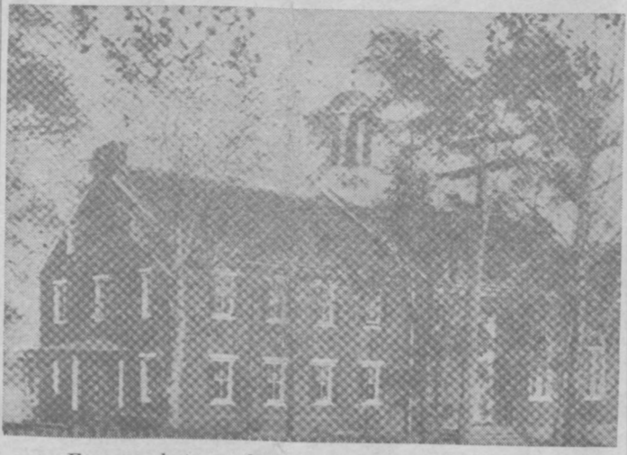
From a photograph taken in 1905. The present Huebener Memorial was built of wood-burnt brick in 1797-98. The present church, also of wood-burnt brick, erected in 1822.
