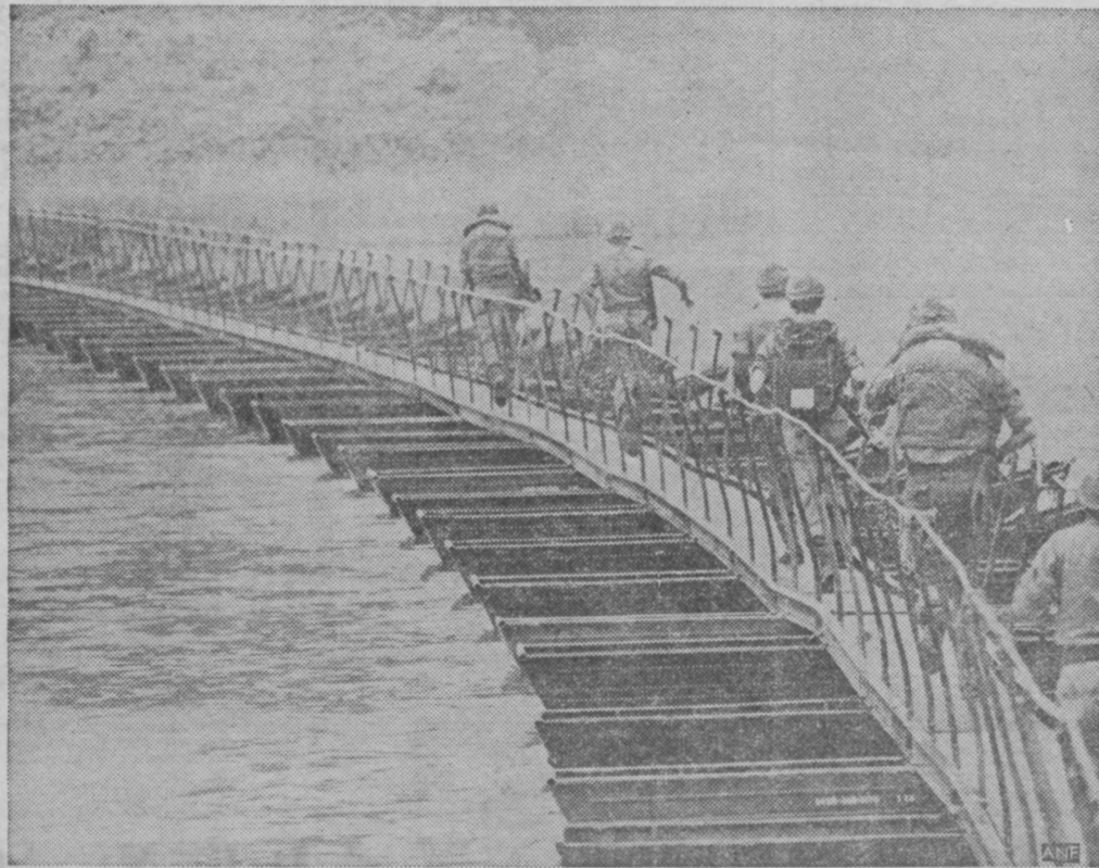
NEW BRIDGE—Soldiers cross the Chattahoochee River during a demonstration at Ft. Benning, Ga. The footbridge was constructed by a crew of Third Army Engineers in just seven minutes. The footbridge assembly was part of a river-crossing demonstration at The Infantry School. (U.S. Army Photo by SFC Jim Stuhler)
