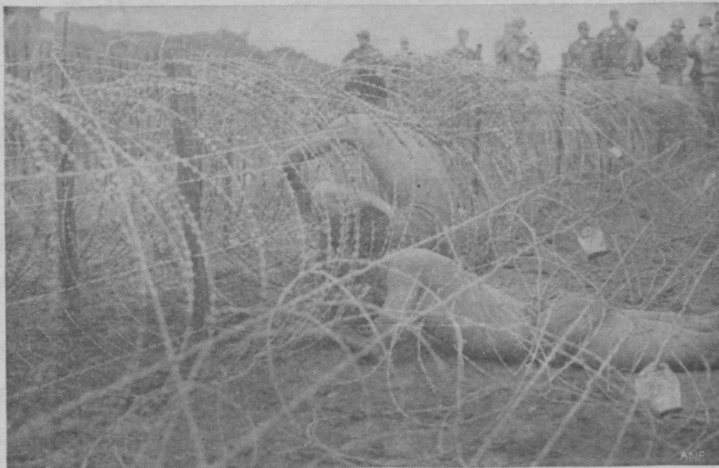
UNDER THE WIRE—Vietnamese soldiers attempt to infiltrate through concertina wire during testing of new techniques for stringing wire obstacles. The obstruction was designed and erected by the 26th Engineer Battalion of the American Division near Chu Lai, Republic of Vietnam. Tin cans attached to the obstacle sound an easily identified warning when jiggled. (U.S. Army Photo by Sp4 J. B. Majerus)
