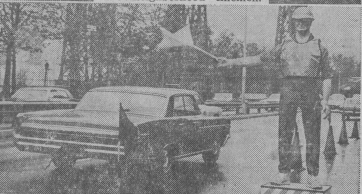
ROBOT TRAFFIC CONTROL — Under watchful eyes of highway engineers, experimental, battery-operated "Silent Sam" directs traffic along road repair section of New York's East River Drive.
