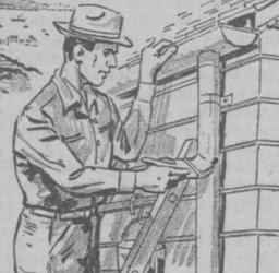
SCIENTIFIC TESTS SHOW IT'S EASY TO PAINT GALVANIZED STEEL IF YOU USE ZINC DUST OR CEMENT-IN-OIL PAINTS.
