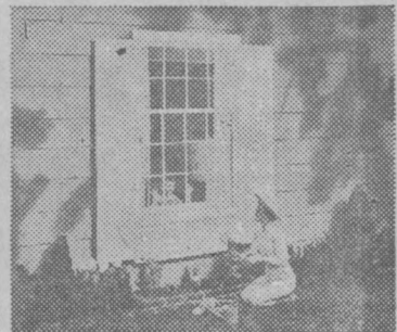
Wide double-hung window of ponderosa pine with its slim mullions and large lower sash is duplicate of an early Amer- ican design, yet is completely modern in function.
