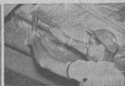
Professor Lund points out that in new construction, batts and blankets of mineral wool can be installed with the vapor barrier down, or toward the unheated side of the floor, if a vapor-barrier type of material is substituted for ordinary building paper between the finished floor and the sub-flooring.
