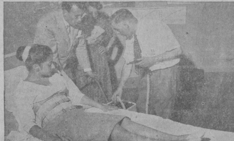
3 Eight years later came the "breathing belt". It compresses and expands patient's diaphragm, offers still more freedom.
