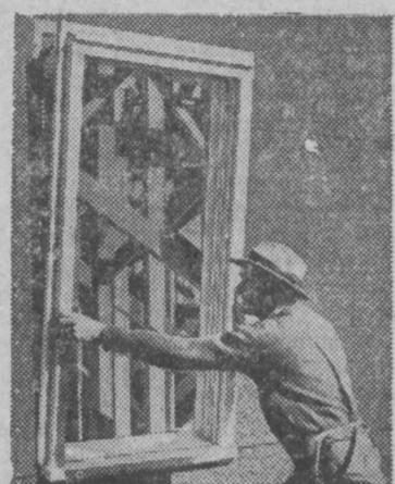
Workman installs window unit of ponderosa pine in wall of new home.
