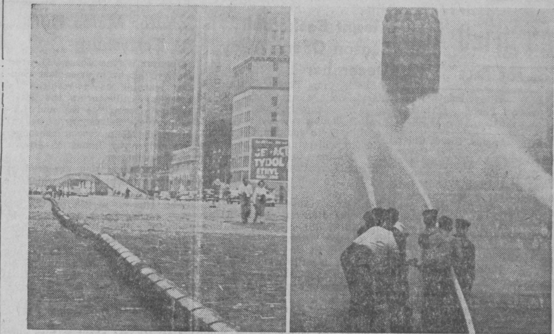
DEMONSTRATION OF PIPE in New York City which can be laid quickly over rough terrain to carry water for fire fighting, city water supply or to pump out flooded areas. This flexible-coupled pipe is stored by the Federal Civil Defense Administration in warehouses throughout the nation for use in emergencies. New couplings allow pipe to be laid without levelling it.
