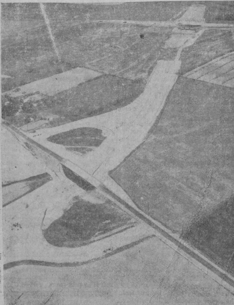
This aerial photo from the Maryland State Roads Commission shows a section of the Frederick By-Pass under construction. The view looking northeast shows the new bridge carrying Cemetery Drive over the By-Pass and its connecting ramps. In the upper right is its junction with U. S. 240 where a new bridge has been built.
