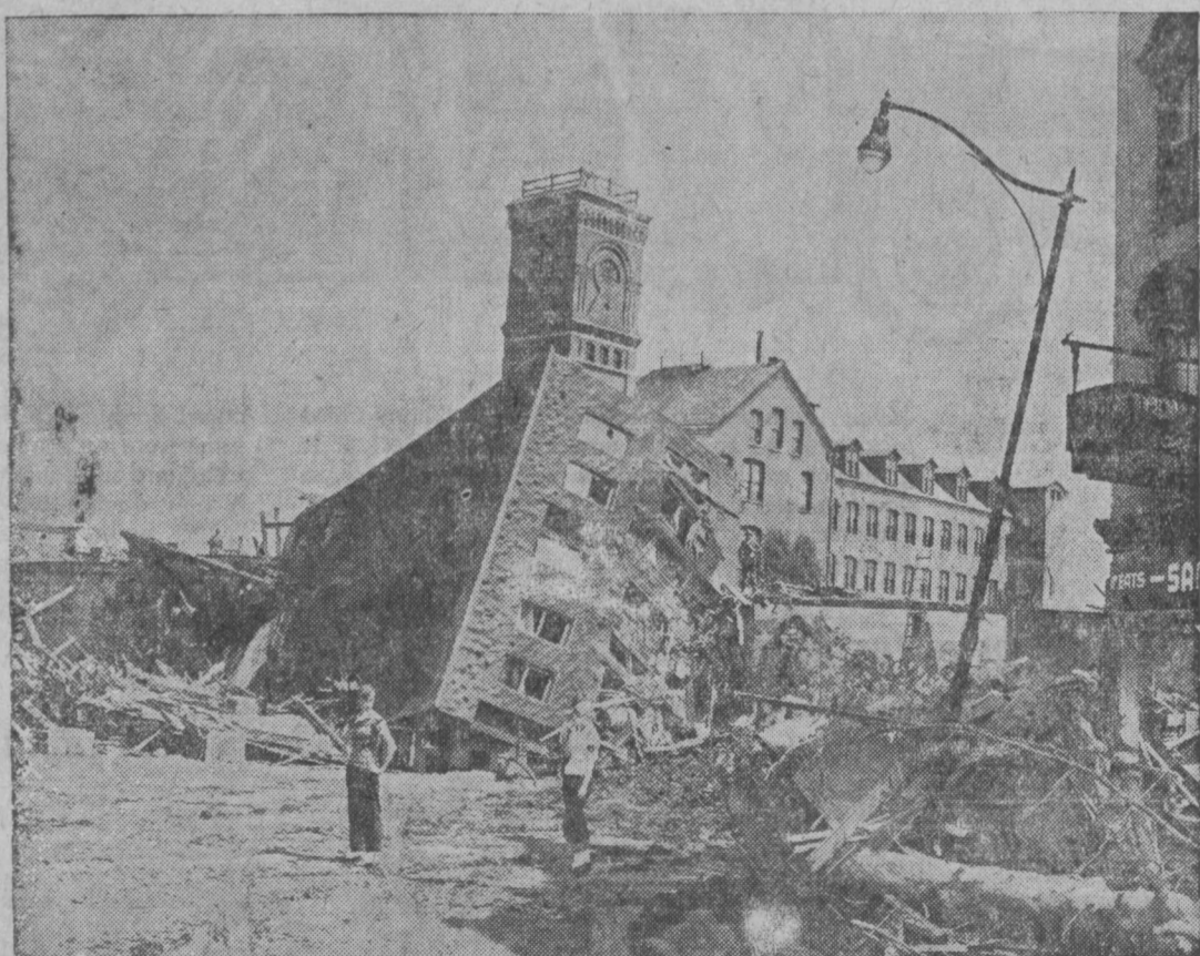
CRUSHED AND BROKEN, this 16-family apartment house in Waterbury, Conn., was left high and dry after the rampaging Naugatuck River receded August 21. This was a sample of devastation in the flood which, according to the Red Cross, destroyed 1,326 houses and badly damaged 4,808. (Wide World Photo)
