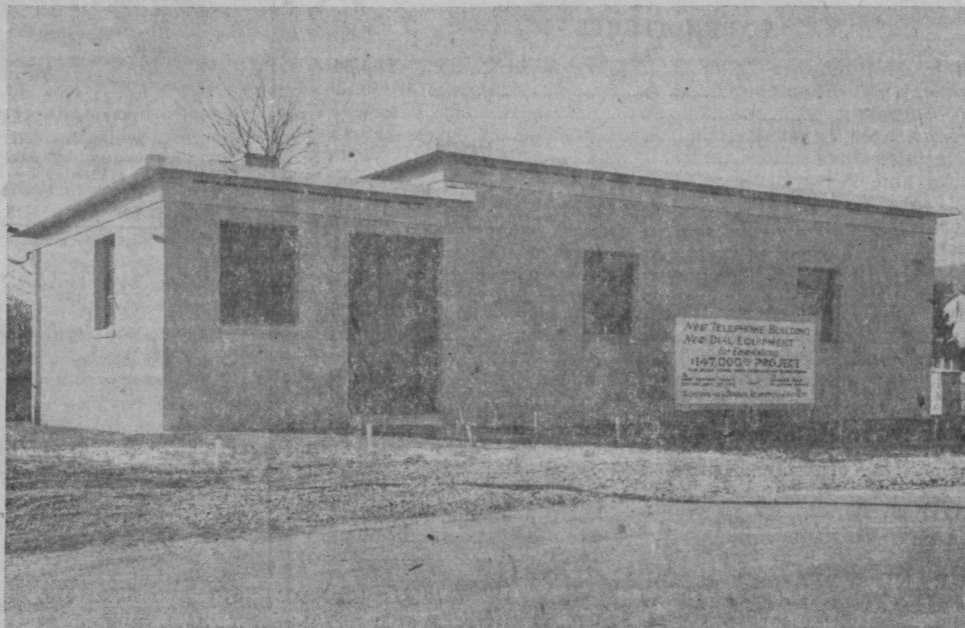
Pictured above is the new telephone exchange building which houses the intricate dialing mechanism. Of concrete block construction, the building is located at the intersection of Chesapeake Ave. and Potomac St. An "open house" will be held Thursday and Friday, Feb. 4 and 5, to which the public is invited. Over 200 school children already have witnessed the "brain" of the dial equipment in action. Dial service will be inaugurated in Emmitsburg next Wednesday morning.
