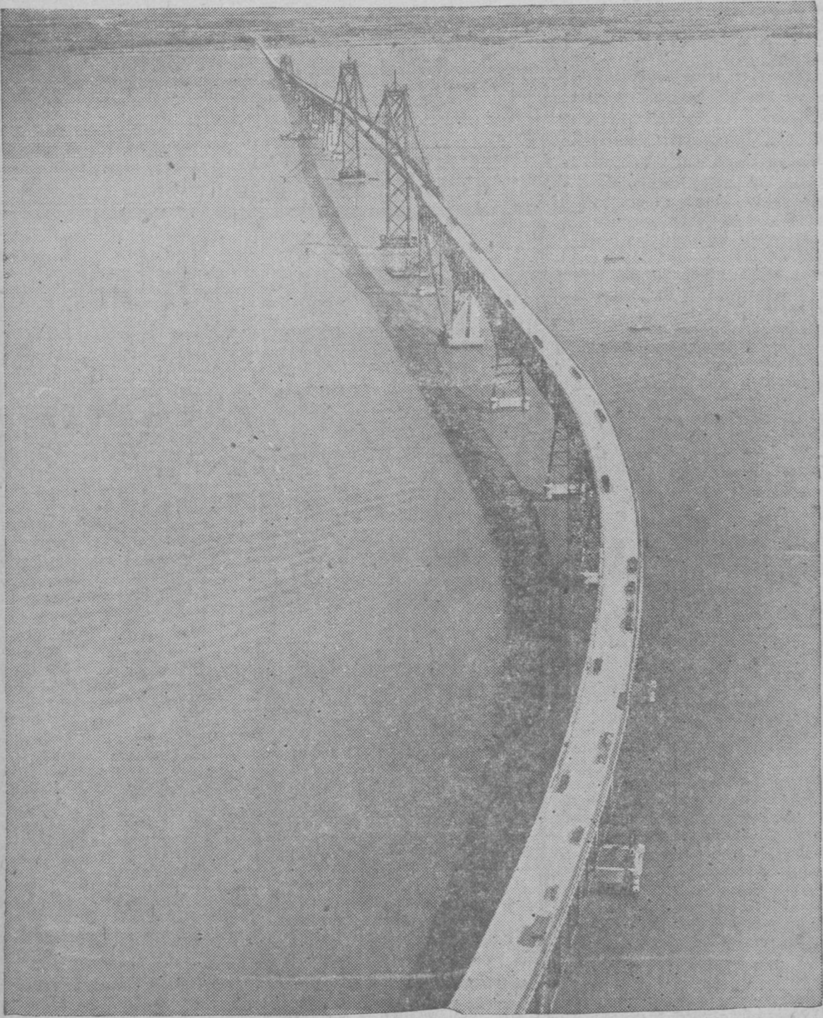
Here's how Maryland's new $44 million Chesapeake Bay Bridge will look from the air when it is opened to traffic later this summer. This photo from the Maryland State Roads Commission, retouched to show the pavement as completed and with vehicles moving over it, provides a west-to-east view of the graceful, four-mile long structure, from a point near the Anne Arundel County shoreline. The two bridge towers mark the boundaries of the main channel. In the distance the new dual highway built to serve bridge traffic can be seen winding across Kent Island, in Queen Anne's County.
