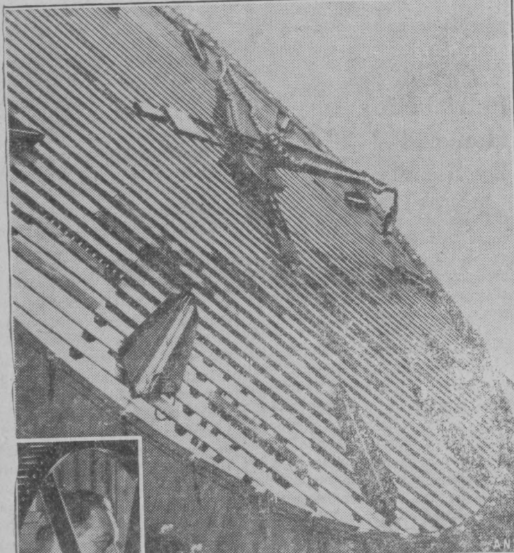
Harold Scheer is one of the few people who always has plenty of time—for he is custodian of the world's largest clock (which is perched atop the Colgate-Palmolive-Peet plant in Jersey City, N.J.) and masters 150 other smaller timepieces throughout the company. Colgate's "King of Clocks" pictured is 50 feet in diameter with a minute hand that travels at a rate of nearly 3/4 of a mile in a 24-hour day. The tiny dot between 3 and 4 o'clock is a workman who is only about half an hour tall. Thousands of commuters, ferry boat captains, tourists and most of the Hudson River traffic and New York City shore line depend on the big clock to keep them posted on the correct time. Scheer, (at lower left) is examining the mechanism behind the clock.
