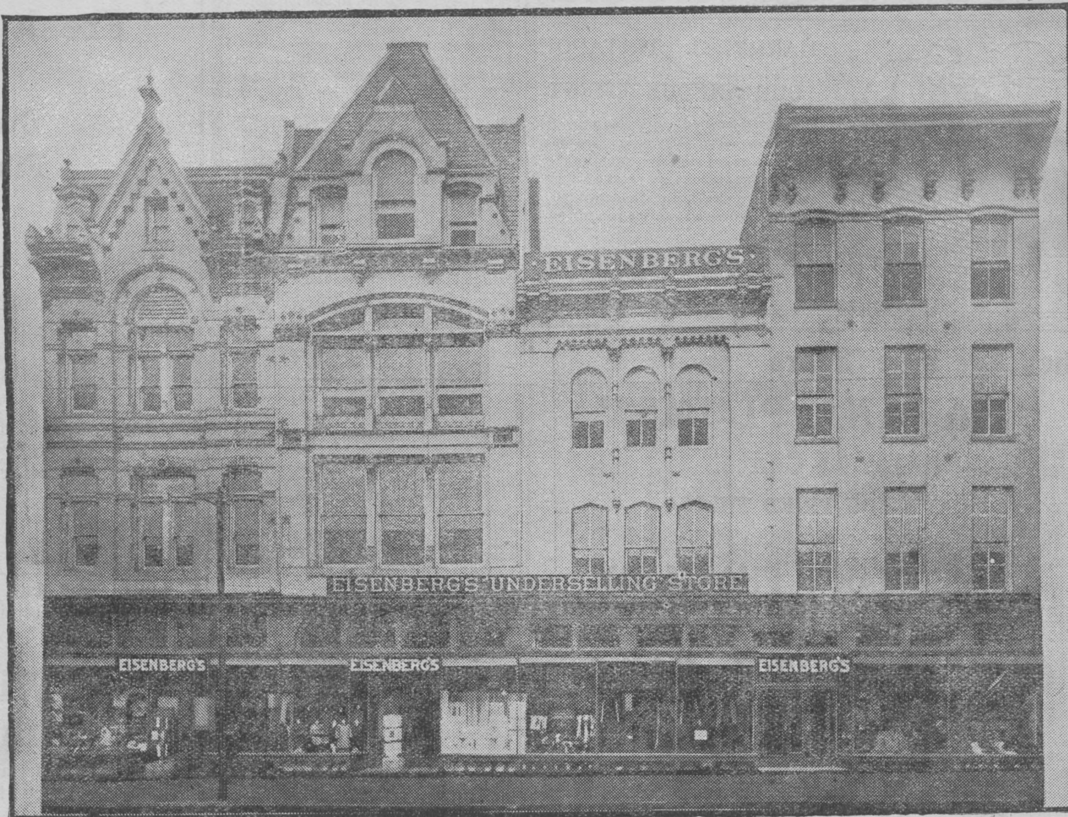
The Eisenberg "Underselling" Store of Baltimore
