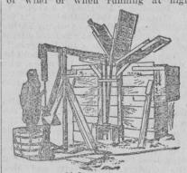
A \$1.50 WINDMILL. speed. A weight should be fastened to one of the fans to balance the weight to some extent of the plunger of the pump; how heavy it should be can best be determined by trial. Mine is about 1 pound; the well being about 26 feet deep does not take much power
