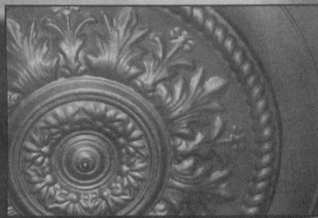
Detail of the theater's new pressed metal ceiling.
