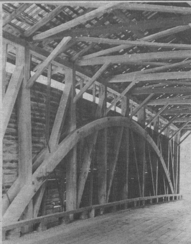
Interior of Jack's Mountain Road Covered Bridge in Carroll Valley. Note the Burr trusses designed and patented by Theodore Burr in 1817. Photo courtesy Debra Brownley
