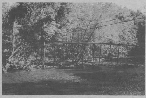
Structure of FourPoints Bridge damaged in flooding caused by Hurricane Fran Photo courtesy of Paul Beale
