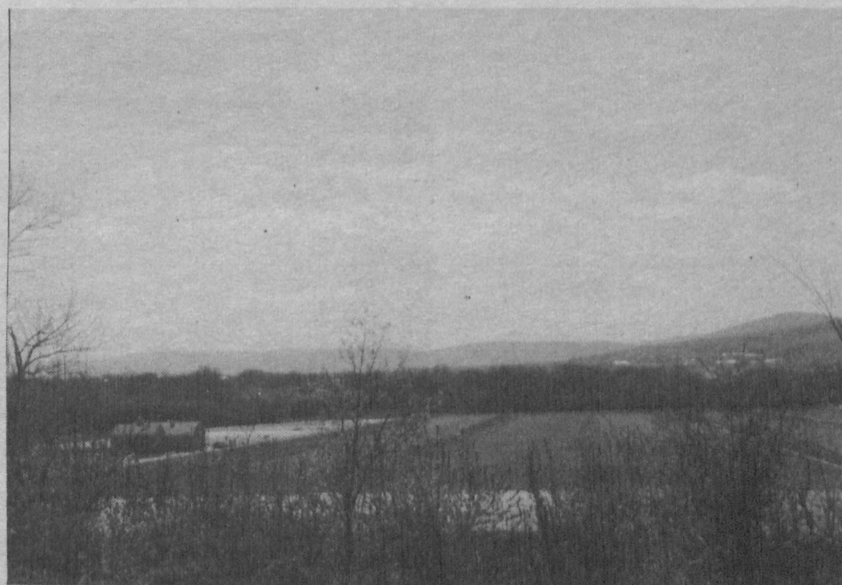
The Emmitsburg wastewater treatment plant.
