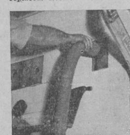
Pieces of siding are removed at intervals along outside wall so that workman can be certain each stud space is compactly filled with insulation. When the job is done, holes in sheathing are sealed and siding is carefully replaced, as it was before.
