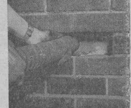
Working from outside the house, workman removes brick and forces mineral wool under air pressure into wall through hole cut in sheathing. Hole is later sealed and brick neatly replaced. Result: warm house
