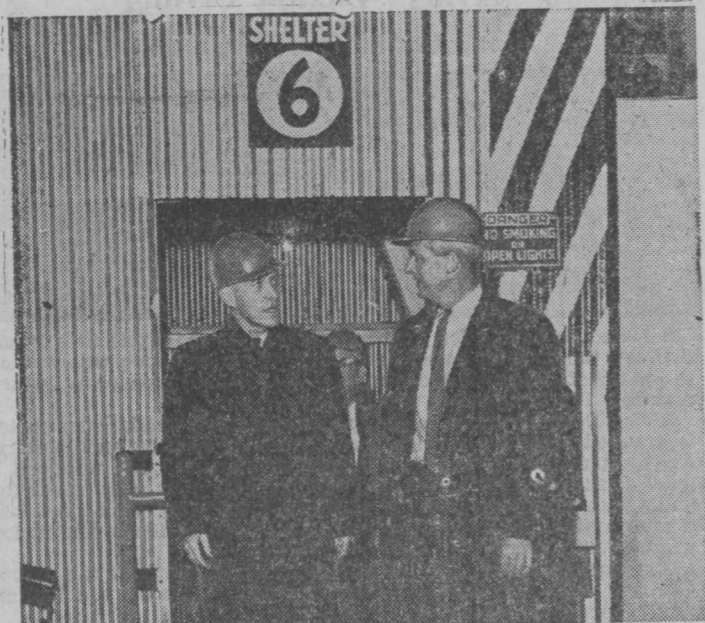
INDUSTRIAL DEFENSE exercise conducted by the Jones & Laughlin Steel Corp. in one of its Pittsburgh plants featured evacuation to shelters of all 2,000 employees in a well-rehearsed routine. The firm, like some other large companies, has a well-developed emergency plan including shelters, first aid training, a relocation site for management and vital records, and fire-fighting. Shown inspecting the plant during the exercise is Leo A. Hoegh (left), director of the Office of Civil and Defense Mobilization, and Dr. Richard Gerstell, Pennsylvania Civil Defense director. (OCDM Photo)
