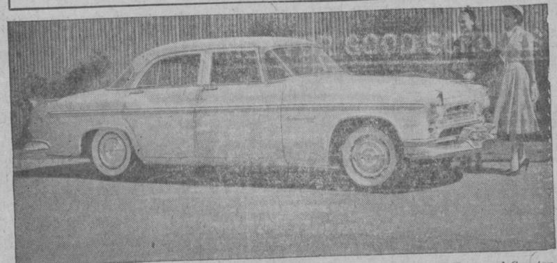
The completely new 1955 Chrysler Windsor Deluxe offers new exterior and interior color combinations, high styling and a completely new 188-horsepower V-8 engine for top performance. In addition to the six-passenger sedan shown, models include the Nassau hardtop coupe, Newport hardtop, convertible and Town and Country wagon on a 126-inch wheelbase. Windsor Deluxe interiors in thirty-three color combinations, feature dramatic new shades that harmonize with or match exterior colors.
