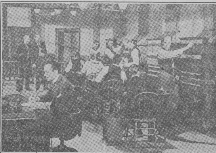
This scene from "Heritage For Victory," shows the original Bell switchboard room in Boston in 1881. "Board men" stood before the panels and switched calls as directed by the "talkers" who, seated at desks, conversed with subscribers. A supervising operator, in foreground, exercised control over the somewhat confusing procedure and waited on any prospective subscriber who chanced to wander into the office.
