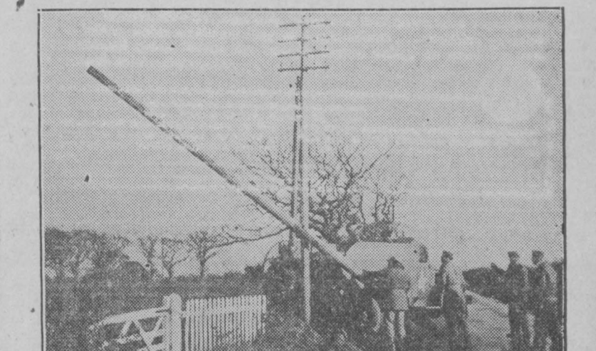
These 8th Air Force Service Command signal construction men in Britain make the job of setting poles look easy. The upright pole is being replaced by the new one being hoisted into position.
