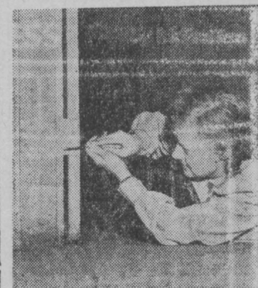
Wherever there are doors children will swing on them, hence the sag. Photo demonstrates the method of prying the screwdriver in taking the sag out of a door.
