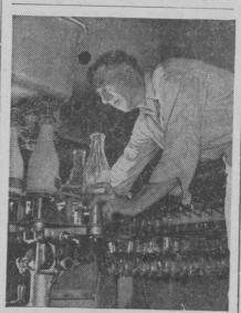
Filling bottles with milk from a mechanical bottle filler.
