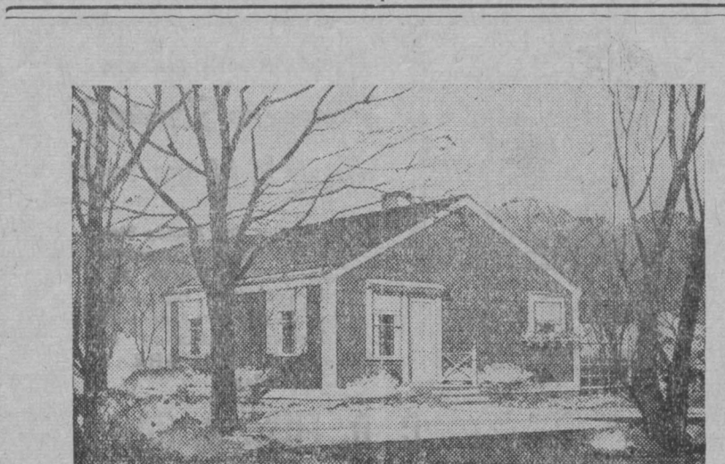
CAREFULLY PLANNED. The four rooms of this northern village house designed by the National Homes Foundation are separated with a minimum of partitions. As shown here, the exterior is of shingles over plywood sheathing; interior is plywood.
