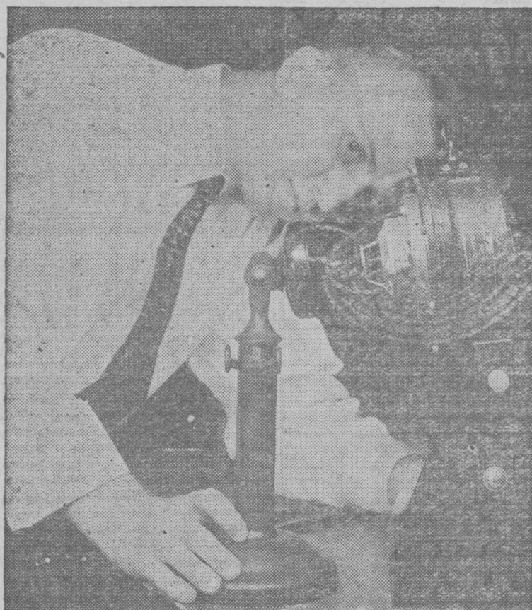
Frederick West of the Bell Telephone Laboratories listens to the speech of the artificial mouth in testing the telephone transmitter. This apparatus is utilized in testing about 1,000,000 transmitters annually.
