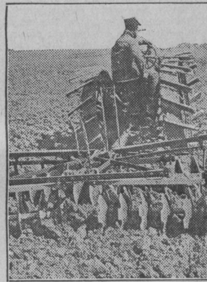
Farm Tractor Drawing Double Disk Harrow.
