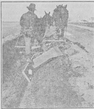
USING "A" SCRAPER IN BUILDING HEAD DITCHES.
