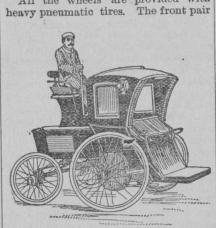
ELECTRIC HANSOM CAB, NEW YORK. is fixed, the cab being steered by the rear wheels. The rear axle is also fixed. But to permit of steering, the rear wheel hubs are hollow and are provided with ball joint journals, so that they move independently of the axle. The side lights are small incandescent lamps, and a lamp is also provided on the inside of
