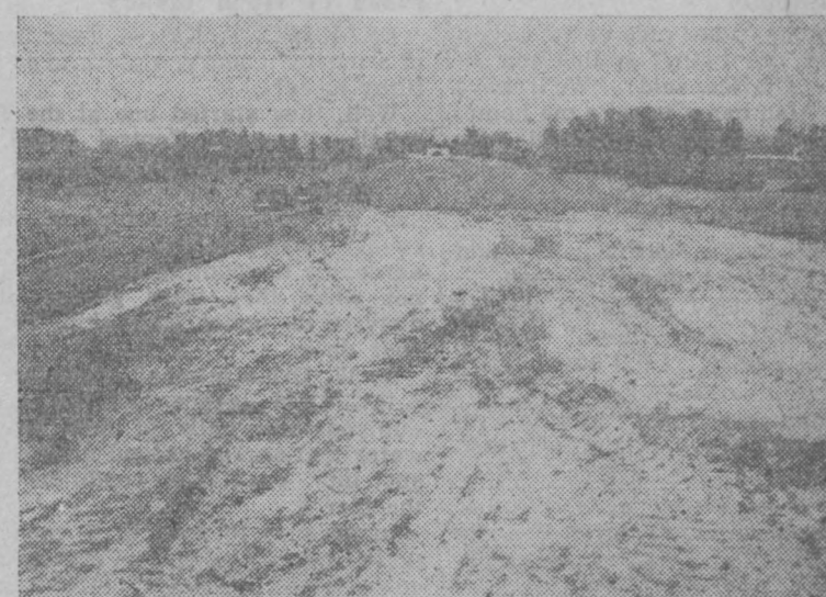
A NEW HIGHWAY TAKES SHAPE —This photo shows the northern portion of the first five mile section of the new Baltimore-Harris Expressway. The building in the middle background stands on the side of Marble Hill Road, where work on the second section of the pressway will begin. The right-of-way width at this point is 200. The highway will consist of two 24-foot lanes separated by a 50-foot area. A contract for surfacing the section of highway shown in photograph was advertised by the State Roads Commission before end of last year.
