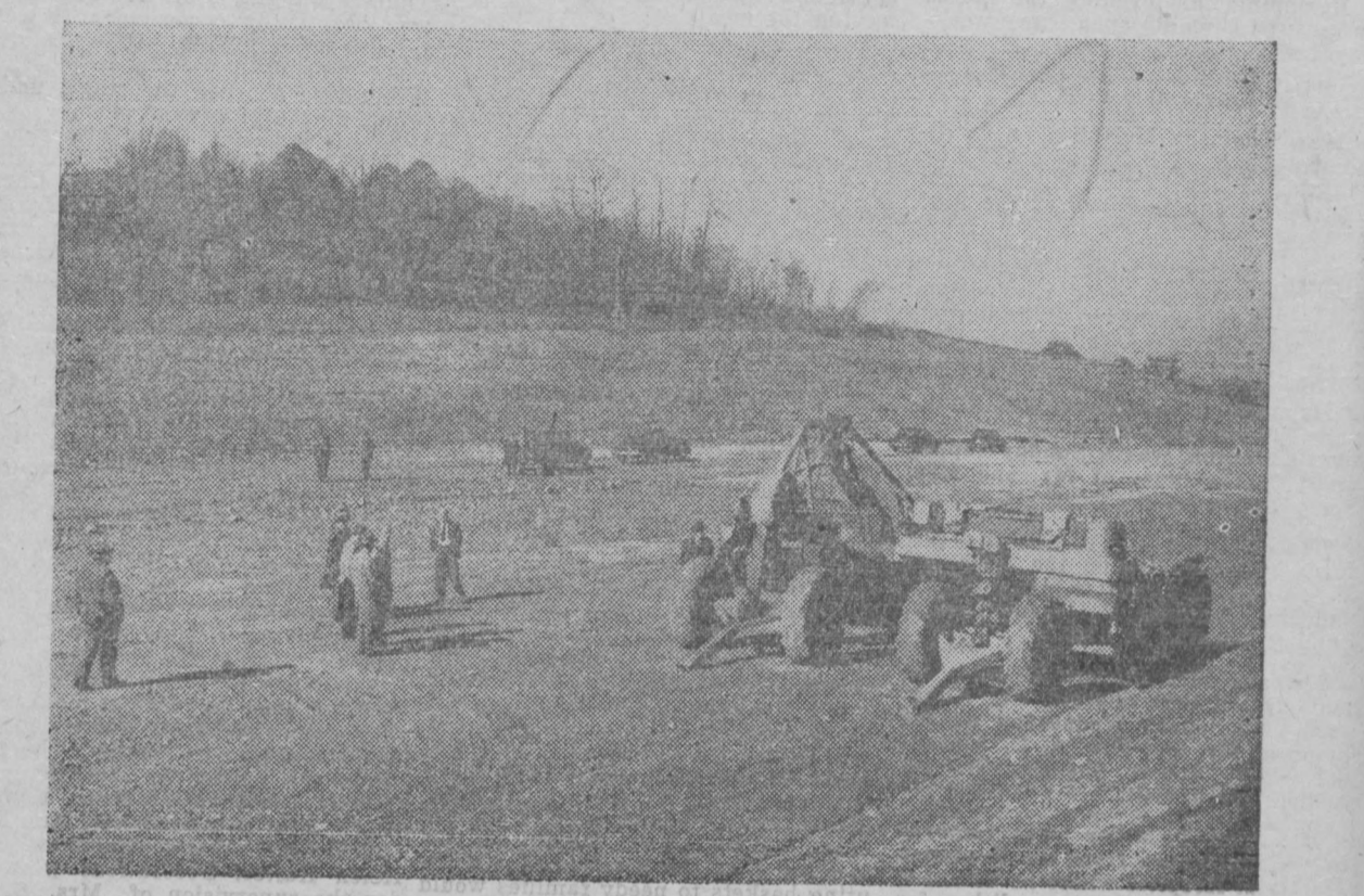
BALTIMORE COUNTY'S NEW EXPRESSWAY—This photograph, made during the recent highway inspection tour of Baltimore, Harford, Carroll, and Howard Counties by newspaper editors and radiomen, shows a section of the new Baltimore-Harrisburg Expressway just north of Padonia Road in Baltimore County. Grading and drainage installations are virtually completed along this first five-mile section of the new highway, and the State Roads Commission plans to ask for bids, before the first of the year, for paving the new road. The expressway will consist of two 24-foot lanes separated by a 50-foot park area.
