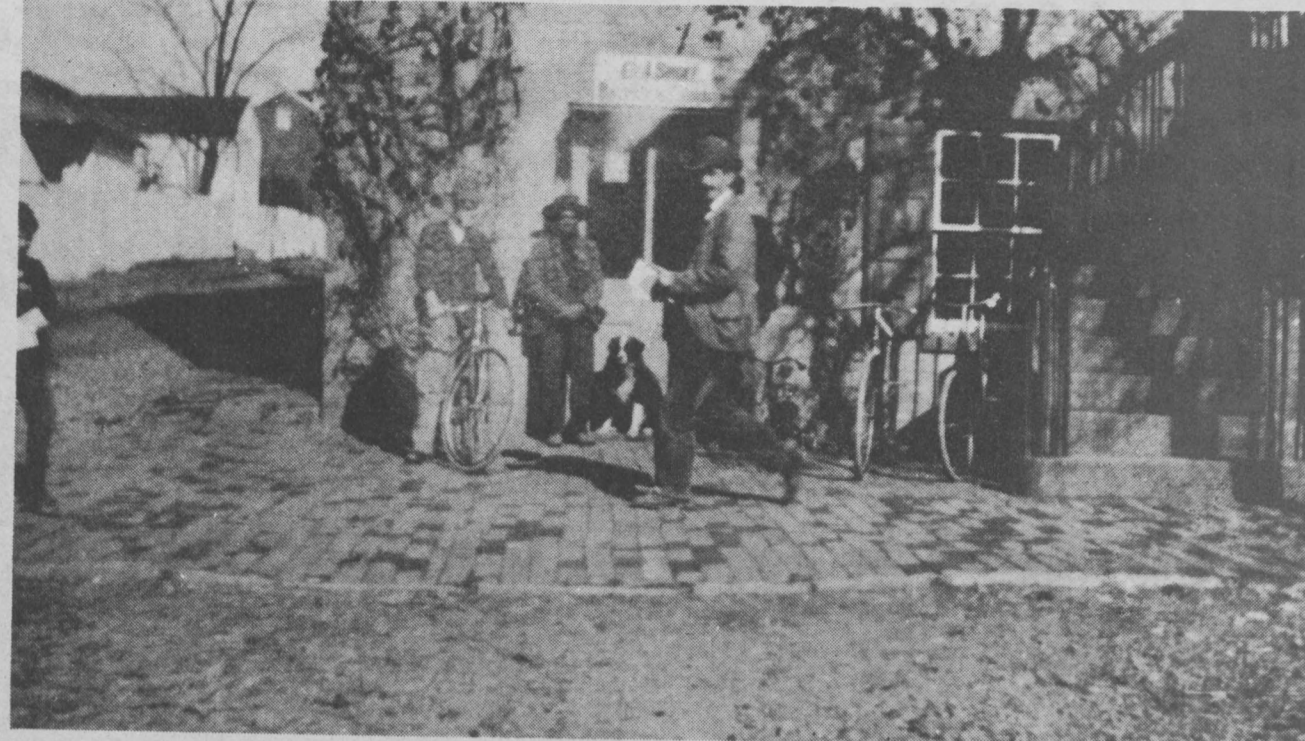
The picture shows the C. J. Shuff Bicycle Shop in Emmitsburg about 1910. On the same site is Houck's Store offering a varied brand of merchandise to the community. The old steps are still standing although the building
