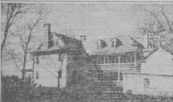
Side view of the Nester House showing rear addition, porches and tenant house.
