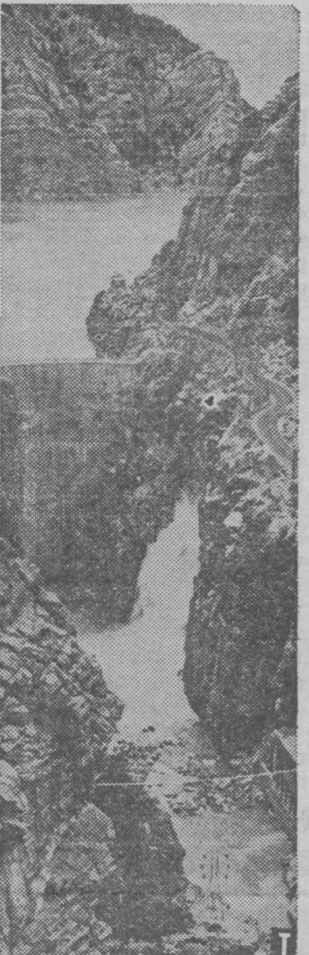
The Buffalo Bill Dam, near Cody, Wyoming.
