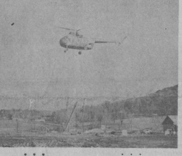
Photo shows helicopter lifting heavy steel standards for the ski lift at Charnita Tuesday. Approximately 20 of these steel poles were lifted by the 'copter, flown up the mountainside and anchored in cement during the day. Officials at the big resort near Emmitsburg, expect to have the ski lift in operation by the
