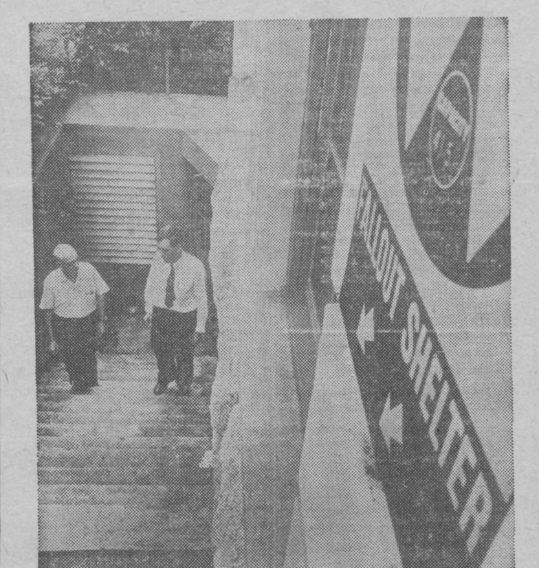
TOWN BENEFACTOR Kenneth W. Pollock (right) of Fort Scott, Kan., emerges from the basement fallout shelter area of the city building where extra ventilating equipment (see vents in background) made it possible to protect about 1,000 persons—many more than could be accommodated otherwise. Using data on the best available local shelter areas in existing structures provided by the Defense Department's National Fallout Shelter Survey, Pollock has spent about $18,000 so far to improve shelters for 6,600, and will go to $50,000 if necessary to improve shelters for the town's 10,000 inhabitants. Money for the project comes from the charity fund of Key Work Clothes, Inc., a local firm which Pollock heads. (Photo by Bill Sneed, Topeka Capital-Journal)
