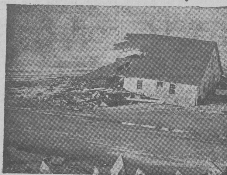
Hurricane-ravaged beach house in Myrtle Beach, S. C., is pushed off foundation, half-wrecked by storm. But wind-resistant roof of asphalt shingles remains in place. Asphalt shingles applied to resist wind are being used increasingly by home owners in areas where high winds prevail. When roof stays in place, interior of house and its contents are protected from deluging rains that usually follow hurricanes and other severe wind storms.
