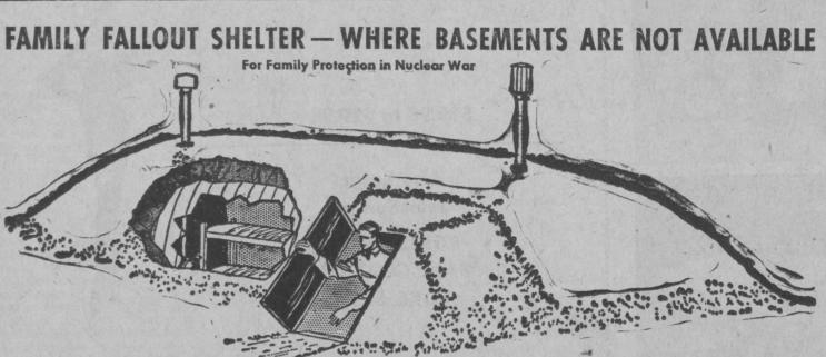
PRE-SHAPED corrugated metal sections or pre-cast concrete can be used for shelters would cost about \$700. A contractor probably would be required to help build it. effective fallout shelters when mounded "The Family Fallout Shelter," published by "ing: Box Home Shelter, Battle Creek, Mich.
