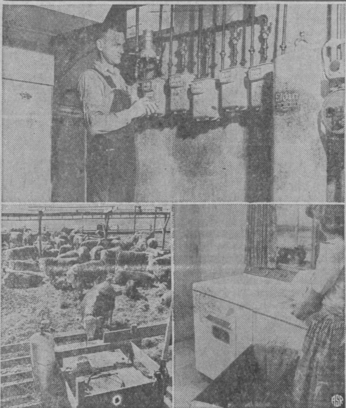
Farmer Raymond Keppy (above) of Scott County, Iowa, reads LP-Gas meters in test to determine operating costs for appliances. Daughter Myrna Keppy (right) prepares load for dryer. LP-Gas is also used for stock tank heating on the Keppy farm (left).
