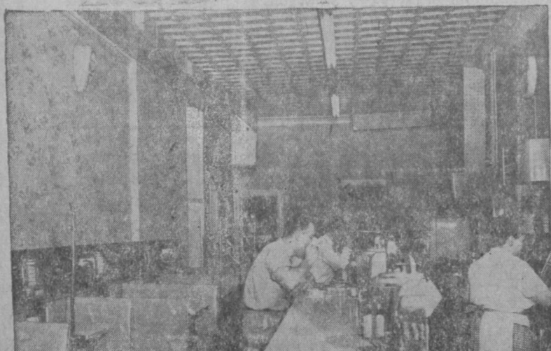
Frick unit air conditioner as installed in The Towne Restaurant
