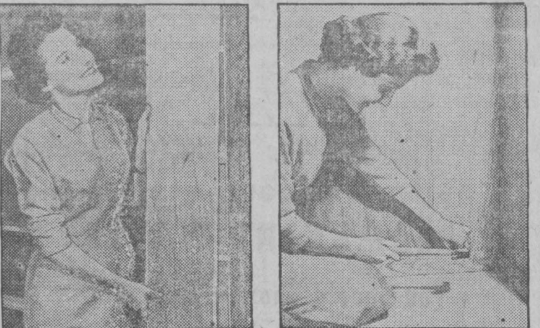
Lock panels firmly to row of clips placed between each two planks. Finish your paneling with moldings and trim of matching Savannah Oak.
