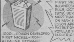
1900—EDISON DEVELOPED FIRST NICKEL-IRON-ALKALINE STORAGE BATTERY. FIRST NON-ACID BATTERY. WORKED 10 YEARS ON IT, MADE 50,000 EXPERIMENTS BEFORE SUCCESS.
