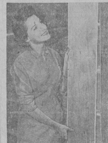
Lock panels firmly to row of clips placed between each two planks.
