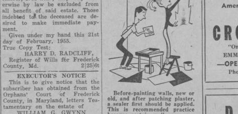
because certain wall areas are invariably more porous than others. If not sealed, they will absorb oil from the wall paint in varying degrees, producing an uneven appearance. The result is often so unsatisfactory that it is necessary to start from the beginning with a sealing coat. Latest type sealers, based on polyvinyl acetate, and water-
