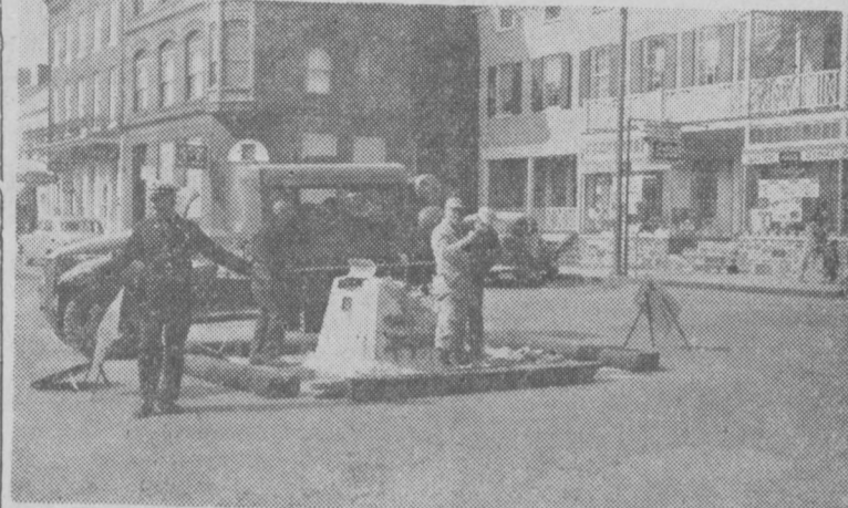
Pictured above are Water Company workmen in the process of removing Square's Blinker which is to be replaced by a traffic light. It took three days to uproot the traffic pylon. The replacement light is expected to be installed in about two weeks.
