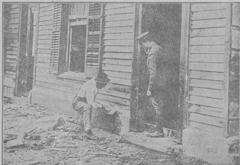
RAT-PROOFING BUILDING WITH CEMENT SIDE WALL.
